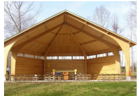
The Apex with Front Bays
